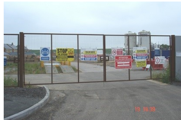
295 Bovis Homes under construction in 2022
