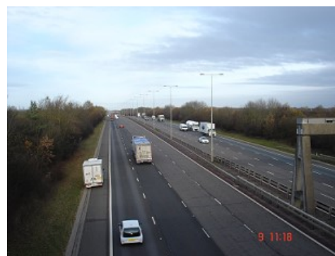
The A1M from St Andrew's Flyover
